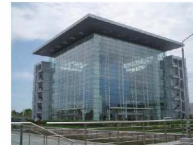
Shanghai Nature Gas Dispatch Center
