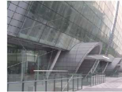
Shenzhen Futian Traffic Control Center
