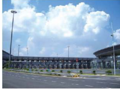
Hong Kong-Shenzhen Western Corridor
