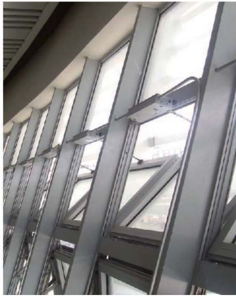
Crank handle GH-388 to the manual bottom hung opening system with 4 windows opening at the same time.
