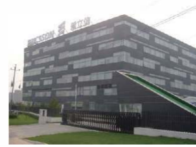
Beijing Ericsson Beijing Building
