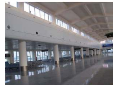
Hainan Meilan International Airport
