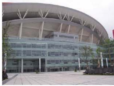
Nanjing Olympia Stadium & Sport Center
