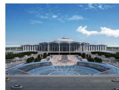
Hohhot East Railway Station Plaza
