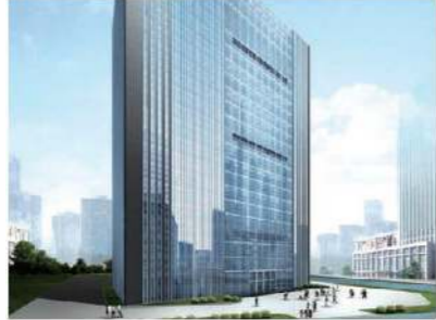
Chengdu Borui Chuangyi Technology Breeding Building
